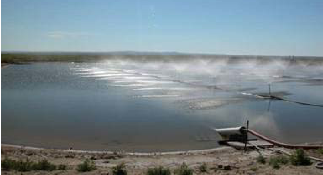
Figure 8-8. Lined evaporation pit in the Battle Creek Field (Montana).
