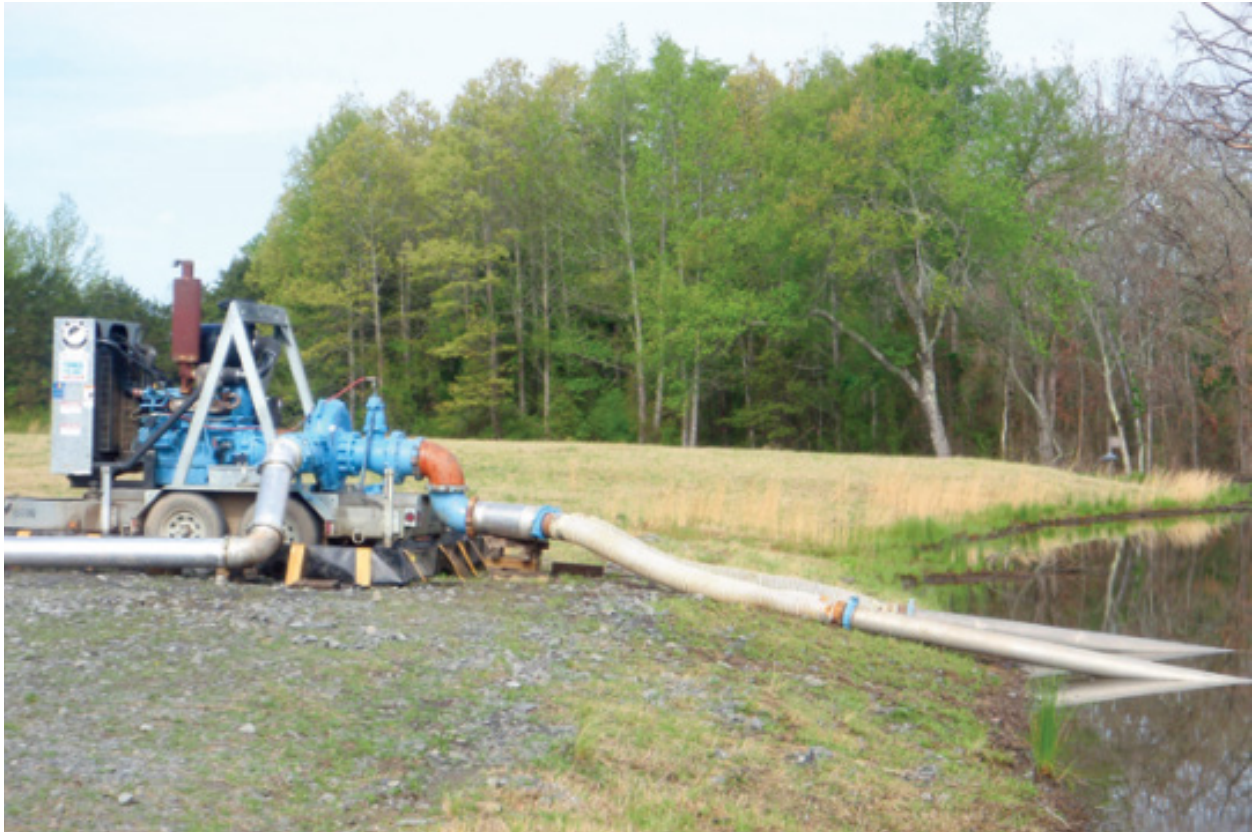
Figure 3-6. Surface water being pumped for oil and gas development.
