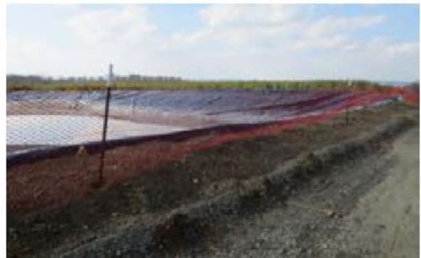
Above: Produced water storage pit. (Source: US EPA) Left: Produced water storage tanks. (Source: US EPA)
