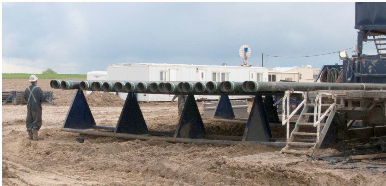
Figure 3-8. Sections of well casing ready for installation at a well site in Colorado.
