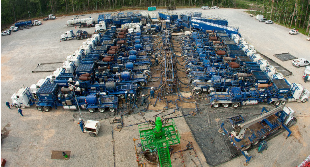
Figure 5-1. Representative hydraulic fracturing site showing equipment used on-site during the chemical mixing process.
