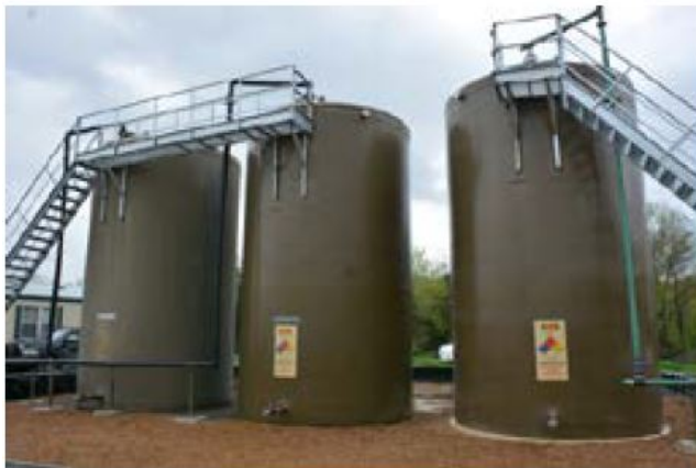
Above: Produced water storage pit. (Source: US EPA) Left: Produced water storage tanks. (Source: US EPA)
